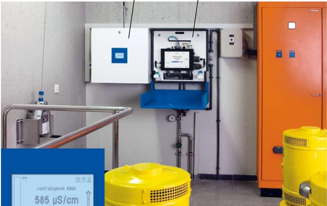
Touch-Screen LCD display with back lighting, with which all parameter values as well as all system information can be displayed numerically and graphically.
